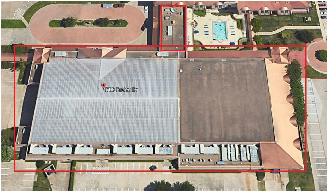
Convention center roof areas in red.
